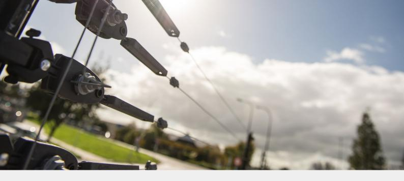
Gallagher monitored pulse fences deliver safe and controlled, energized pulses that last only a millisecond - enough to give a potential intruder a fright and deter them from making a second attempt on the fence.
